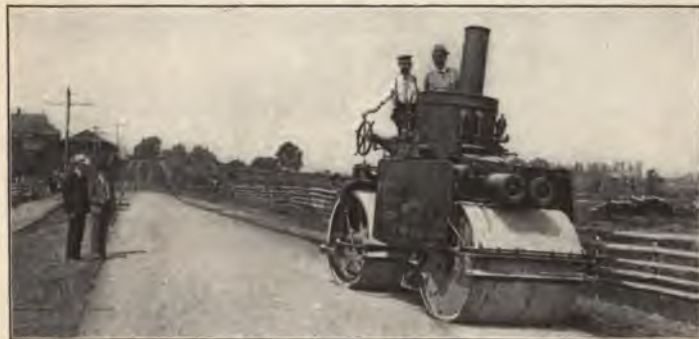
3. Finishing the road.
